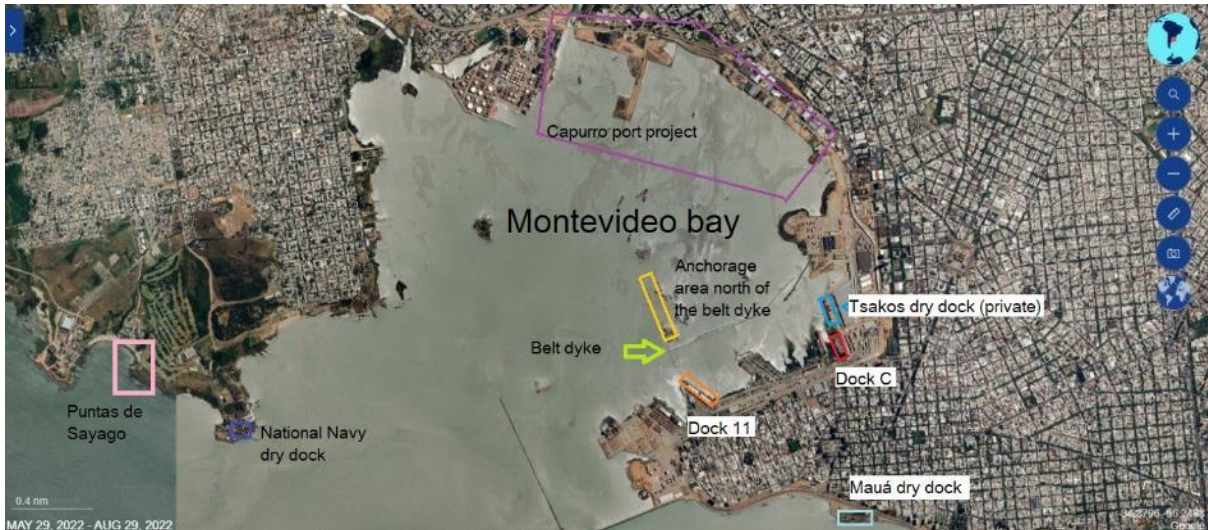
Figure 39: Port of Montevideo. Note that the Tsakos dry dock collapsed in December 2022.
